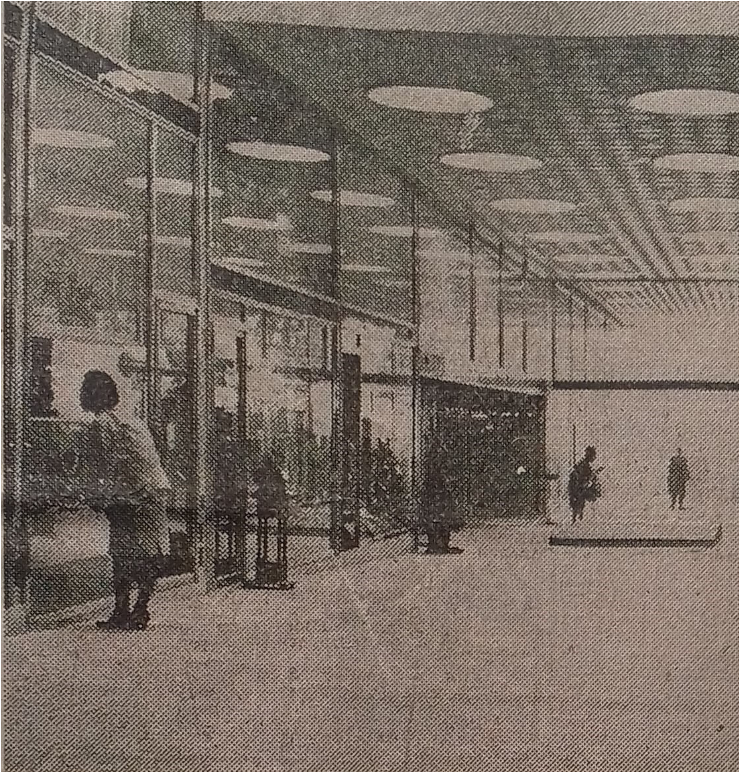
Figure 5 "The Toison d'Or Gallery accessible to pedestrians", La Lanterne, October 8, 1965. © KBR.
