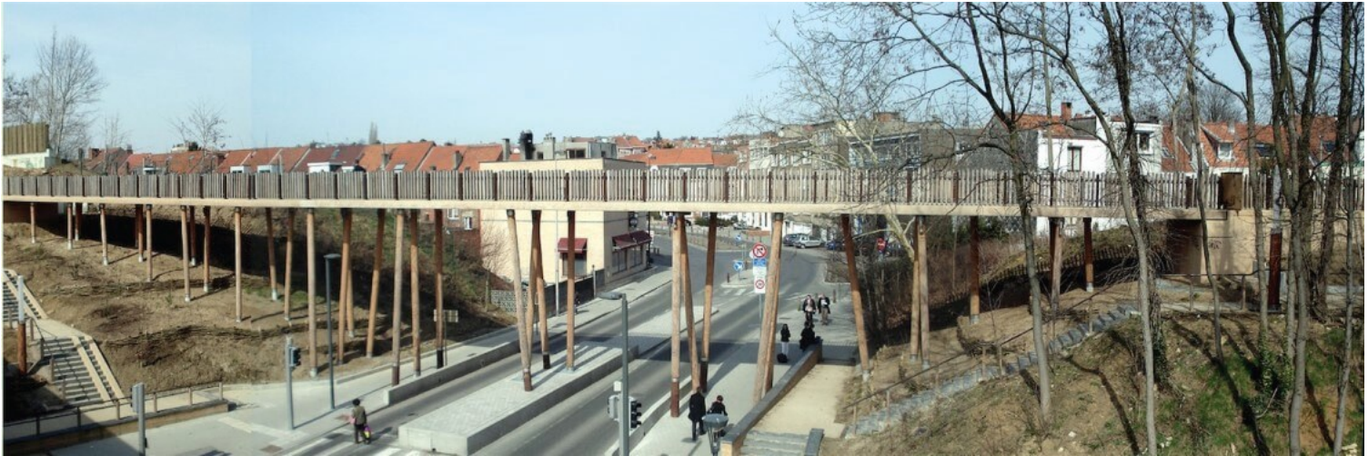
Figure 9 Example of a separate urban cyclo-pedestrian infrastructure, developed along the route of an old railway line located above the street. La Promenade du Chemin de Fer, 2010. © Dessin et Construction.
