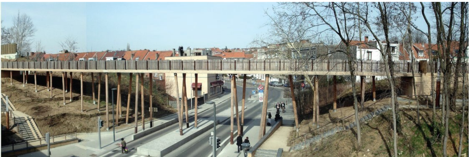
Figure 9 Example of a separate urban cyclo-pedestrian infrastructure, developed along the route of an old railway line located above the street. La Promenade du Chemin de Fer, 2010. © Dessin et Construction.
