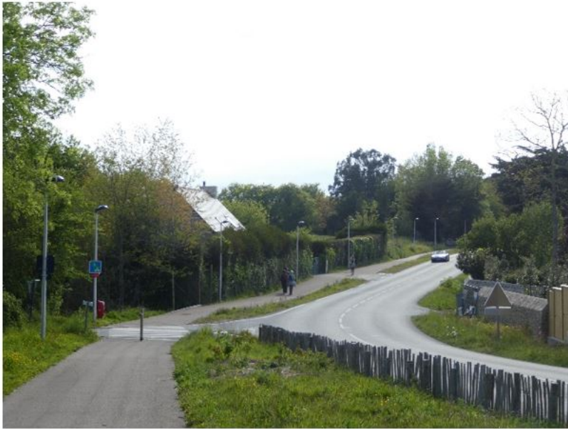
Figure 5: Example of a departmental road that has been adapted to promote and ensure the safety of active mobility: wide cycle way on the side, lit at night, separated from the road and running continuously through villages (Pierre Helwig).
