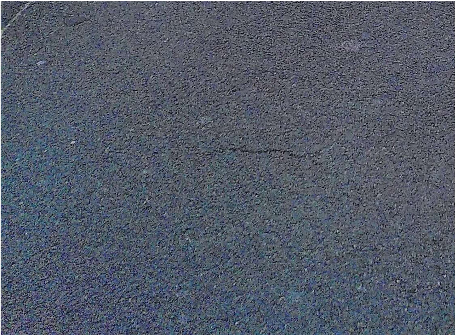
Photograph 7: Avenue Charles Flahault, Montpellier, June 2021, credit Adrien Poisson (researcher)
