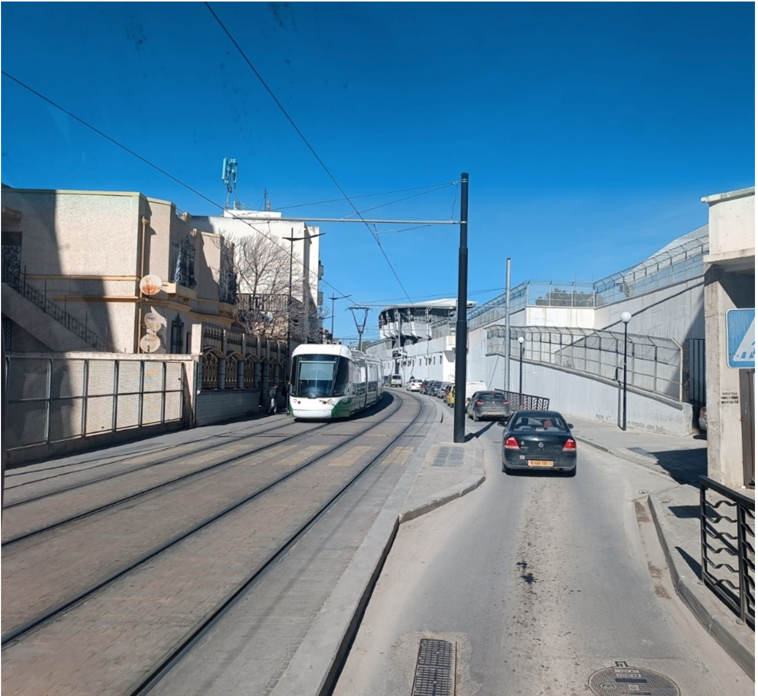
Figure 4: How the tramway and roadway in Constantine occupy public space to the detriment of pedestrians. Photograph by the author.
