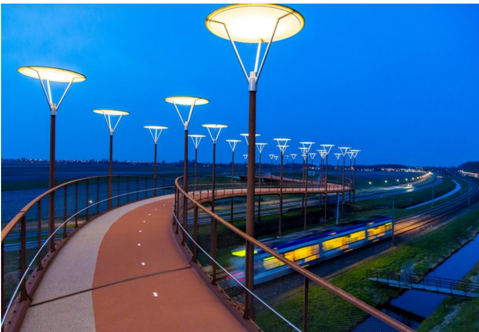
A 220 metre long bike path and footbridge over a highway and railway track, part of a cycle network in the future nature reserve New Driemanspolder in Zoetermeer. Credit: Jochen Tack / Alamy
