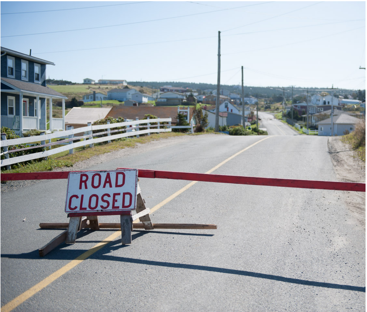
Some roads were washed out entirely, others looked intact but were structurally compromised. More than 100 communities were isolated for up to ten days. Photo: Colin Peddle
